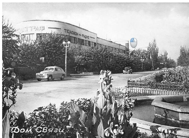
Fig. 5. Communication House - General Post Office
